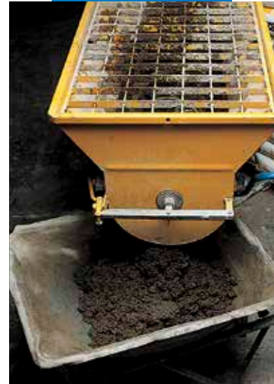
Mixing Mapecem in a mini-batcher
