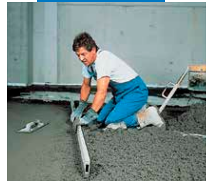
Using the straight-edge
