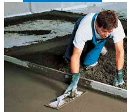
Tamping the Mapecem screed
