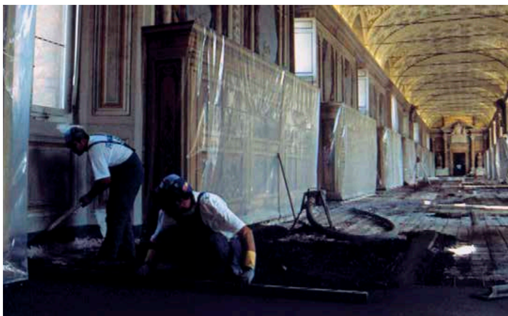
Laying and smoothing of the Mapecem screed - Sistine Halls - Vatican City
