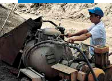
Mixing Mapecem with an automatic pumping unit
