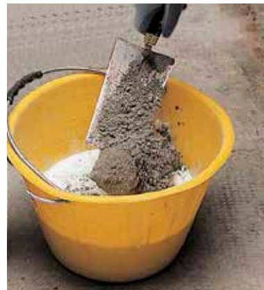
Mixing Mapecem with Planicrete SP to make an anchoring slurry
