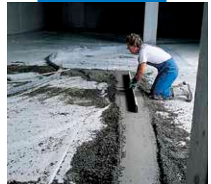
Preparing a levelling strip
