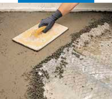
Covering pipes with Mapecem and reinforcement netting
