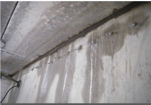
Packers inserted, ready for resin injection to seal leaks
