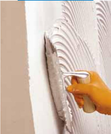
Spreading Tixobond Fine S1 on a substrate
