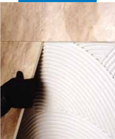
Laying large-sized porcelain tiles on walls
