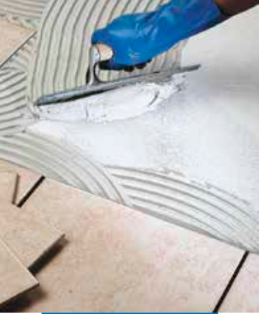
Installation of single-fired tile on floor
