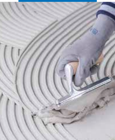
Spreading Adesilex P9
