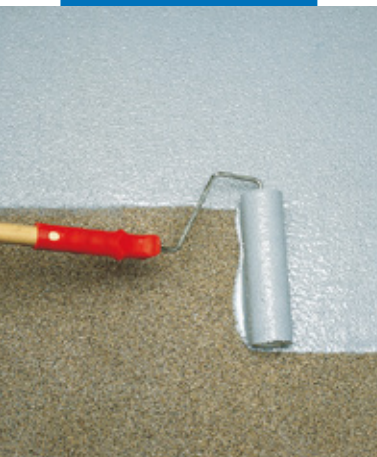
Applying Mapecoat I 24 with roller
