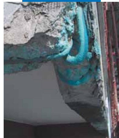
Reinforcing rods of the front side of a balcony treated with Mapefer 1K
