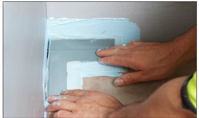
Installing Elastoproof Prefabricated Corners
